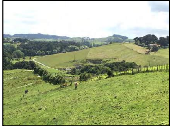
Photo 6: Possible open pit borrow area. Note the failing batters where quarry cuts have over-steepened the slopes.
